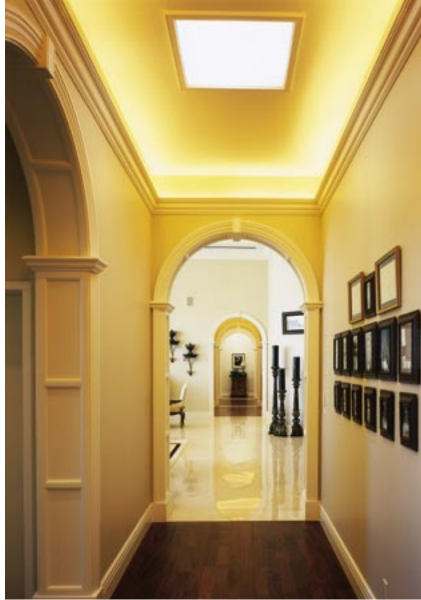
Above: Arches throughout the house were designed to provide a classical accent. Manufactured by Monterey Woodworking, the 13 arches are not all the same size. Three different forms were used for each sized arch. The golden light of the recessed ceiling lights creates intimacy.
